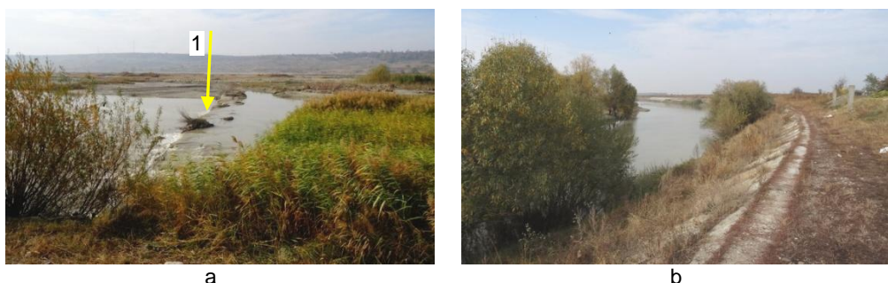
Fig. 4 The state of the "Tupilati-Roman" natural site on the Moldova River: a - bottom (1) in the calibrated riverbed, Pildești area; b - protection of the concrete slab in the Cordun catchments area (year 2018).
