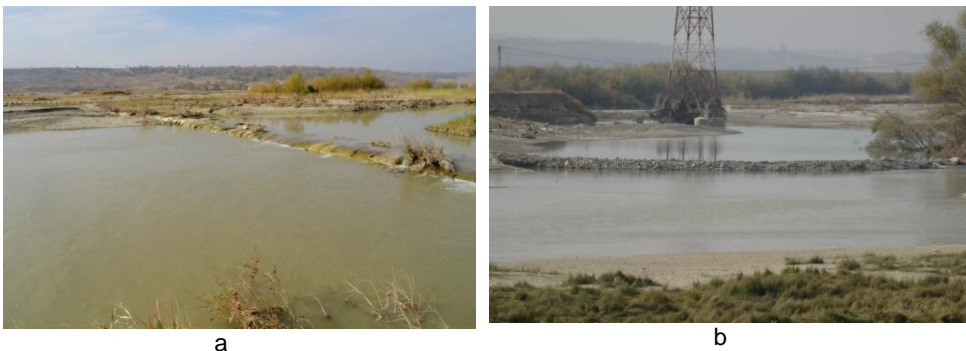
Fig. 7 Degradation of the aquatic habitat through works in the riverbed of Moldova River: a - transverse works (bottom threshold); b - exploitation of the ballast with morphological degradation of the bed (year 2018).
